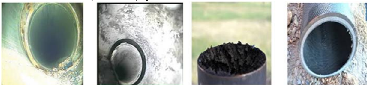
Fig. interior pipe defects
