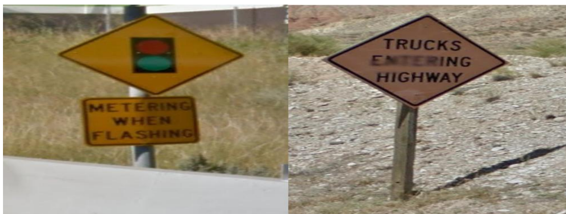
Figure: 1 Example of dirty traffic signs Source: Street view images of Google.
