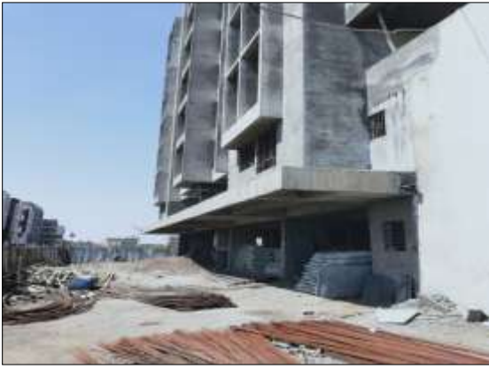
Fig 1: Construction of flat slabs
