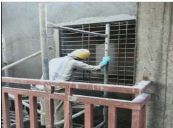
Fig 3 : Safety for labours – helmats, gloves
