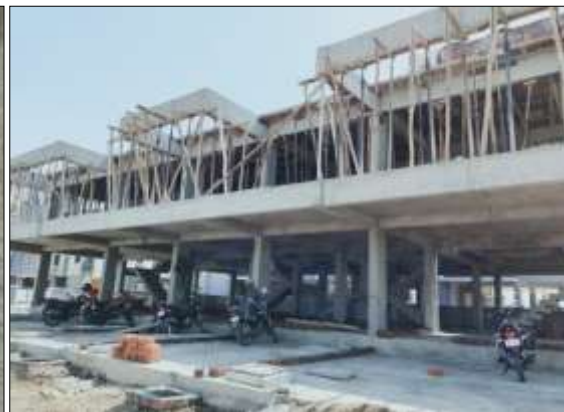
fig 4 : Construction of EPS panels for internal walls
