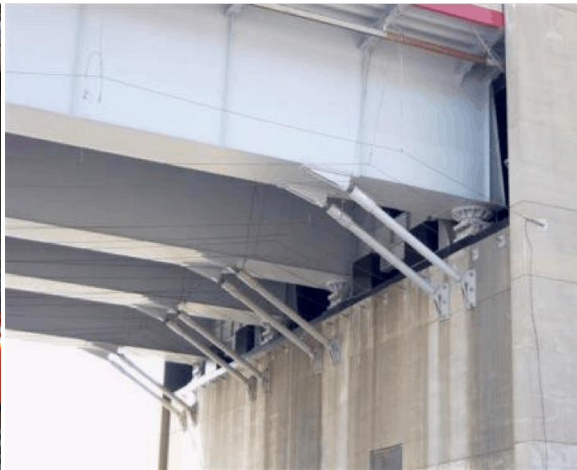
FIG: Viscous damper (For bridges)
