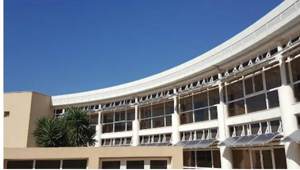
Fig. 4. PV Panels Overhangs, Industrial Research Center Source: (Talal Salem, 2015)
